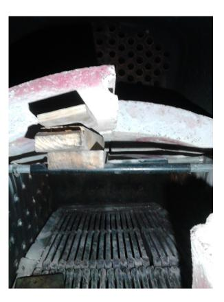
In the left-hand photo, the left wall supporting studs can clearly be seen. These studs are positioned higher at the rear of the fire box and descend at an angle towards the front of the fire box.
